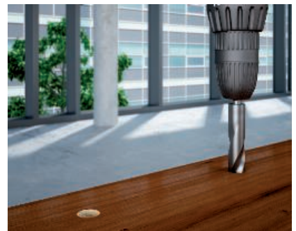
Preparation for fastening stand mounting Drill holes (Ø 16 mm) in the tabletop are required to mount the fastening stands.
