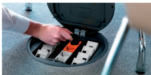
Installation in floor boxes
