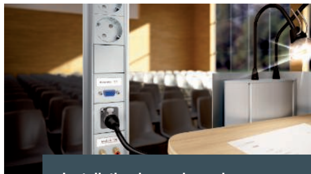
Installation in service poles
